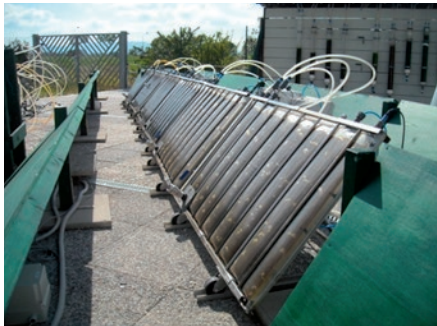
GWP®-III reactors at F&M pilot plant (Florence-Italy)
